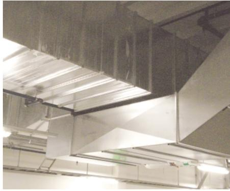
**FIGURE 4.** Cross-creased duct.
