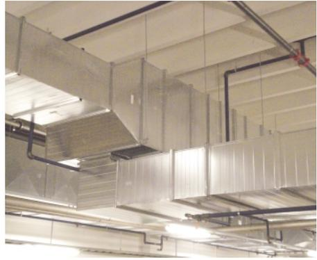
**FIGURE 5.** Transverse-stiffened duct.
