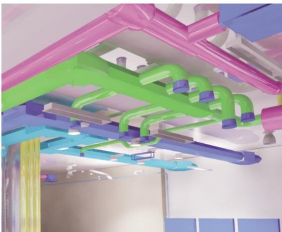
**FIGURE 11.** Colour-coded ducting.
