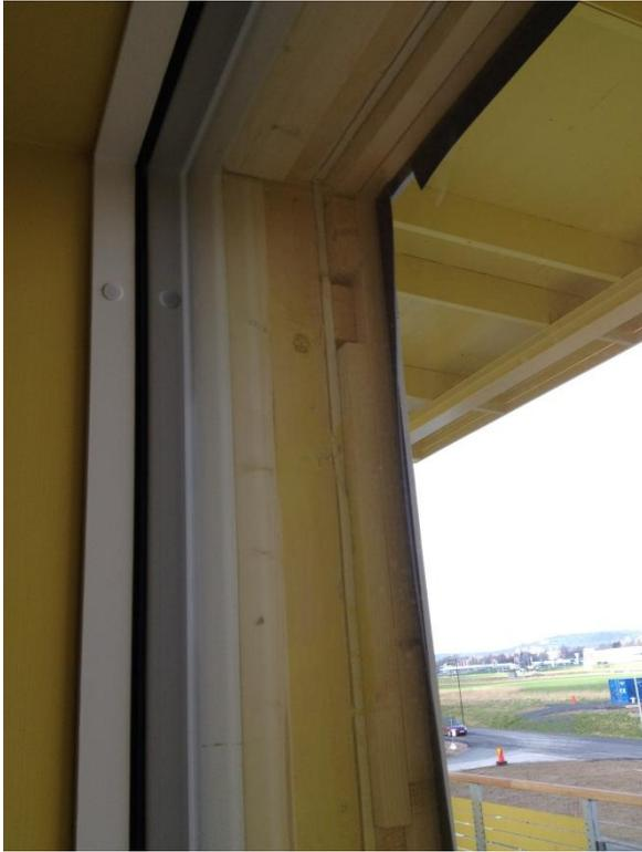
*Figure 3. Window frame with the upper part unfinished*
