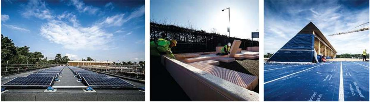
*The building's 480 square metre rooftop solar photovoltaic array; The Isoquick insulated foundation system that eliminates thermal bridging; The Siga Majcoat wind-tight membrane on the roof provides protection from the elements while being breathable*
