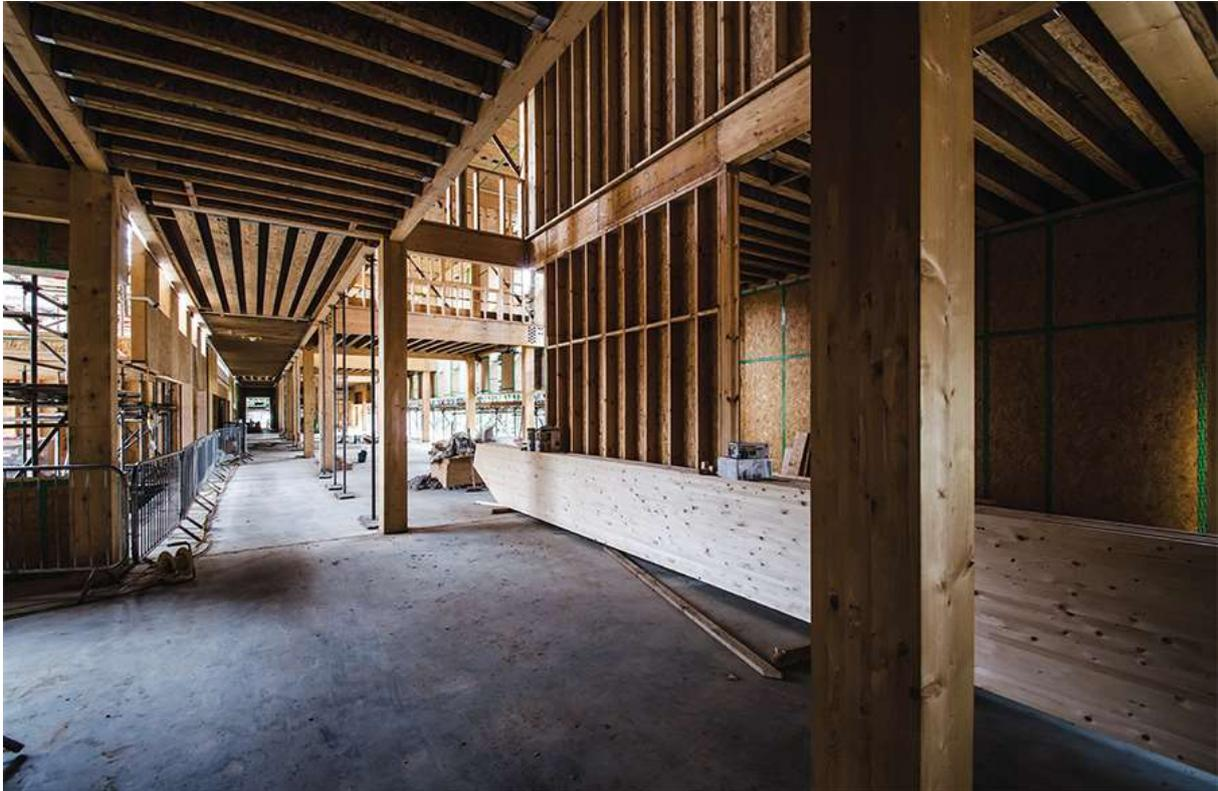
*The Cygnum timber frame structure, primarily made of locally grown pine*
