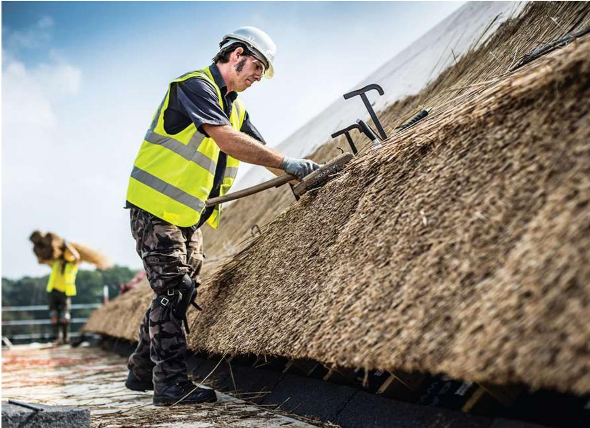
*The thatch cladding is perhaps the most distinctive feature of this building; three hundred panels were manufactured and thatched off-site, and the panels then hooked onto horizontal battens lining the perimeter of the building. The building also features a wide array of other sustainable materials including recycled timber finishes, wood wool acoustic boards, spray-on cellulose, and wall coverings made from hemp, nettle fabric and reeds*
